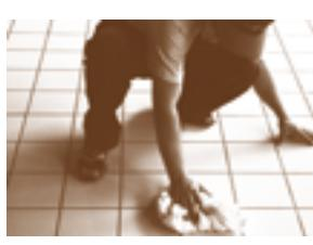
costs limited and speed up maintenance operations, the concentration of the detergent must always be as low as possible. For raised floors we suggest to choose bright or polished surfaces in large sizes: these materials can be dry cleaned or with the minimum use of liquids. After the floor is laid it is necessary to make a very accurate initial cleaning with proper products.
